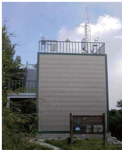
▶ Fully equipped roof of the Mt. Lulin air quality monitoring station
