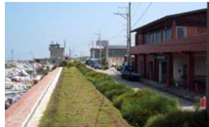
After greening of seawall at Baisi Community, Miaoli County
