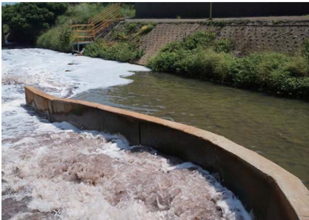
▶ Effluent discharging in Guanyin Industrial Park (觀音工業區)
