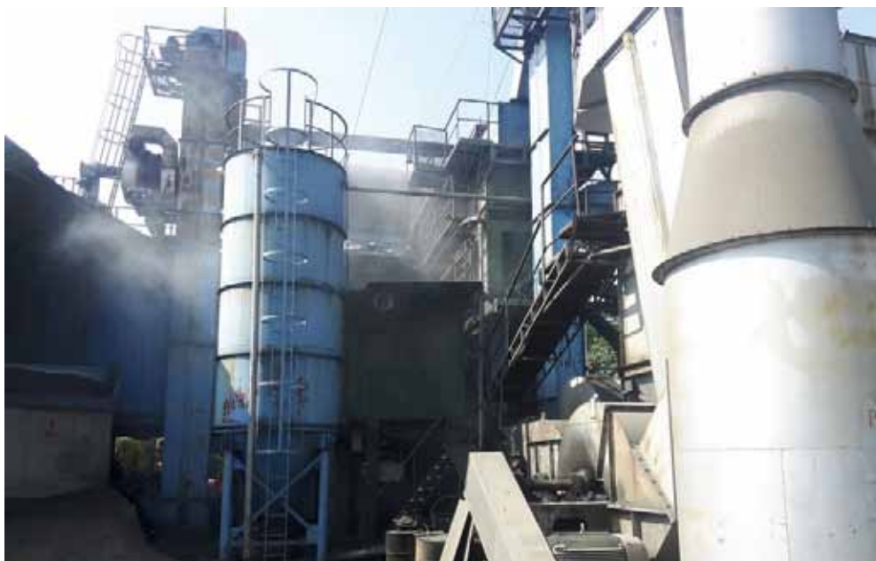
📍 Mixing asphaltic concrete is a major air-polluting act.
