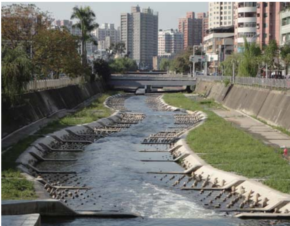
▶ Liuchuan River in Taichung City after remediation
