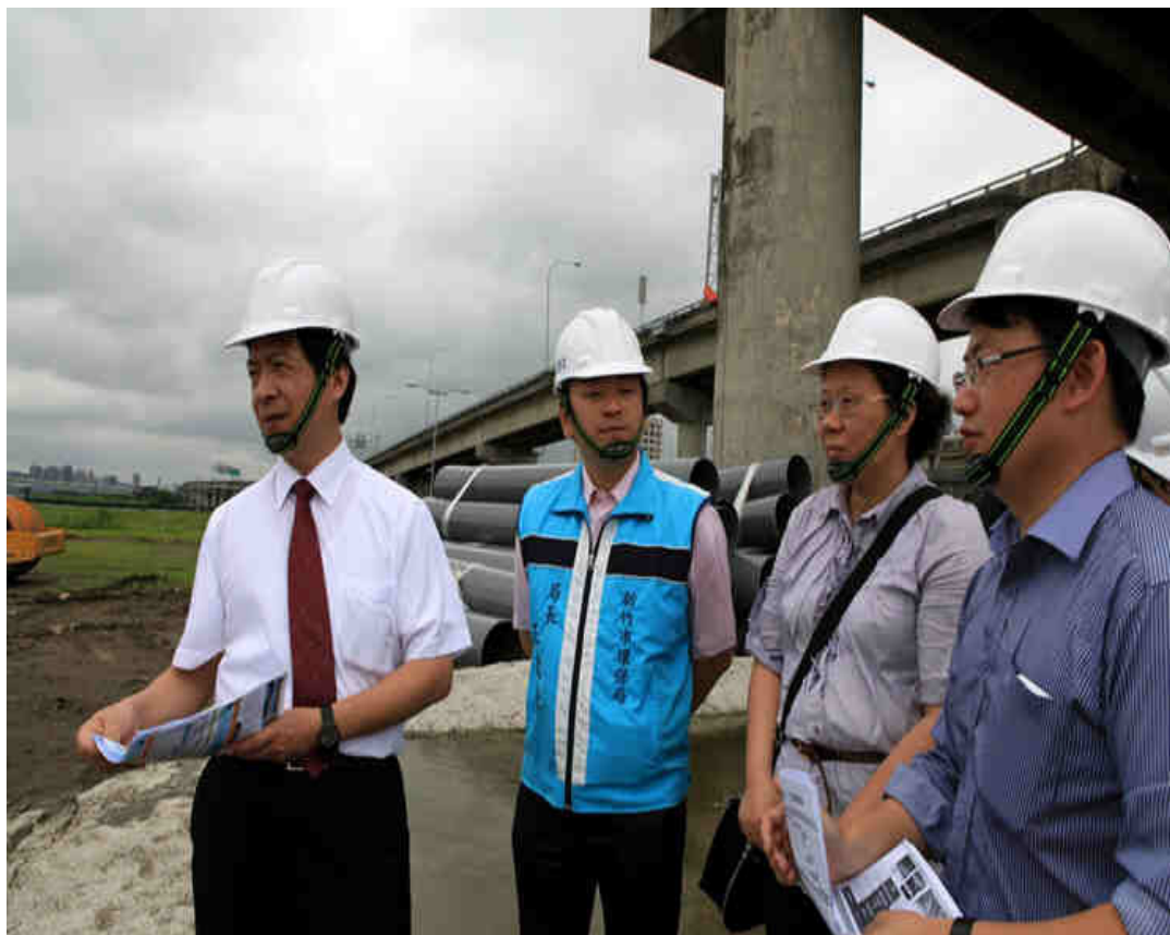
▶ Deputy Minister Shin-Cheng Yeh (left) inspects the wetland construction work on the Touqian River
