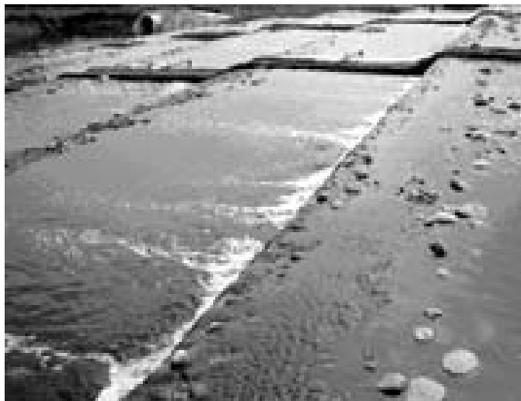
Stone-filled terraces are designed in riverbeds to increase dissolved oxygen (DO) content, filter the water and improve its quality by allowing biological contact oxidation (BCO) treat the water.
